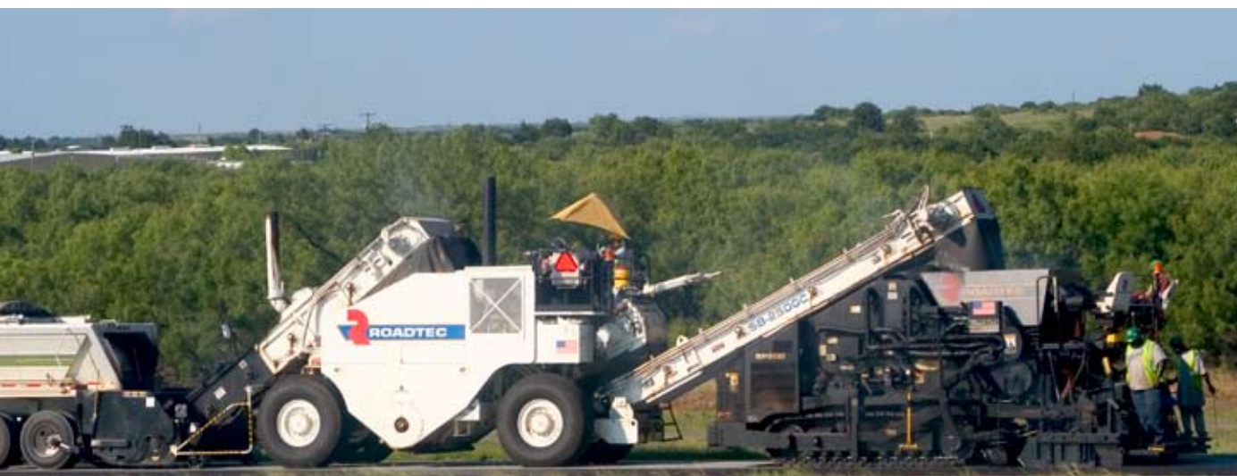
Use of the Shuttle Buggy® material transfer vehicle with the gravity-fed Spray Paver allows crews to pave without stopping and produces smooth, segregation-free pavements in record time.
